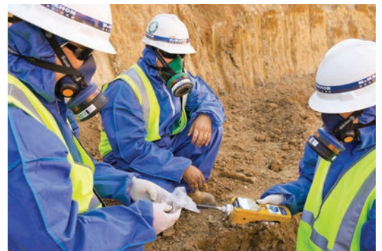
Collecting samples at Hills Industries remediation site
