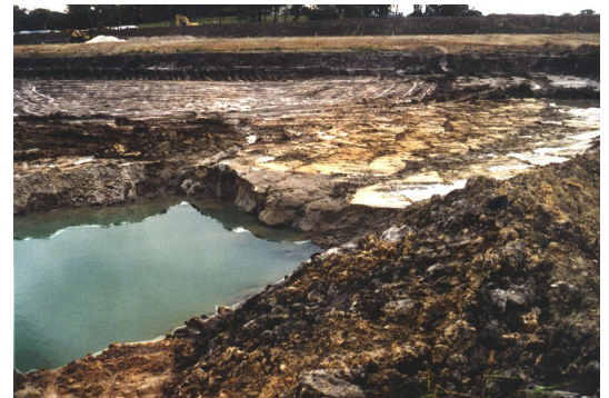
Exposed acid sulphate soil
