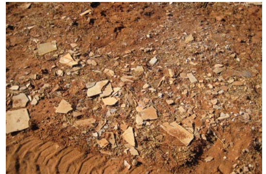
An example of asbestos building materials found on site
