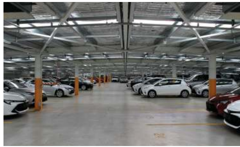
CMI Toyota Vehicle Storage Building Construction Matthews Architects, $3.7 million, Adelaide, SA
