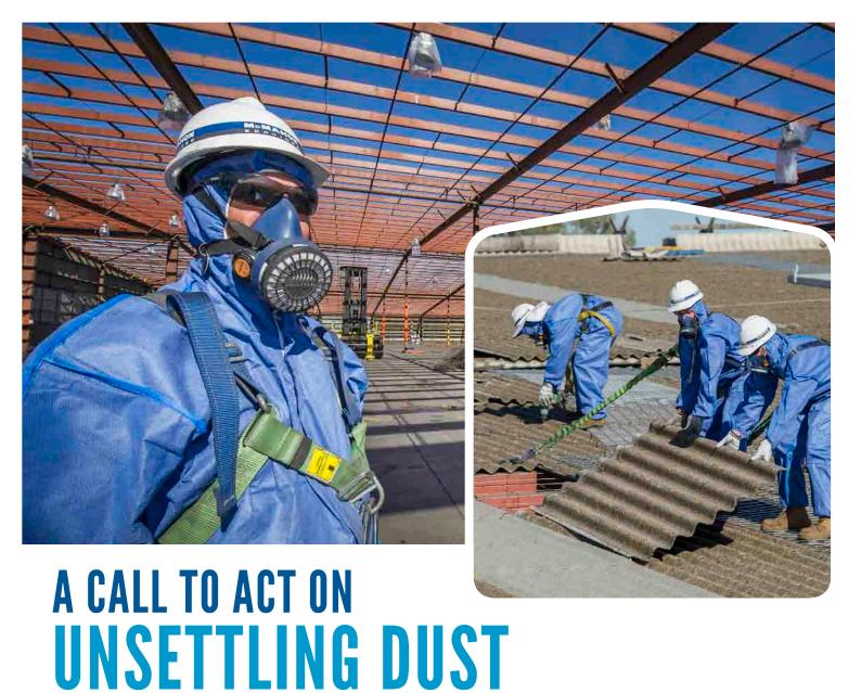
Asbestos dust and debris settling on glass bottles stored in Gillman, South Australia, prompted a quick response to decontaminate the facilities and remove the asbestos roof sheeting and wall cladding.
