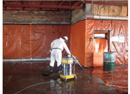
Vacuuming contaminated areas
